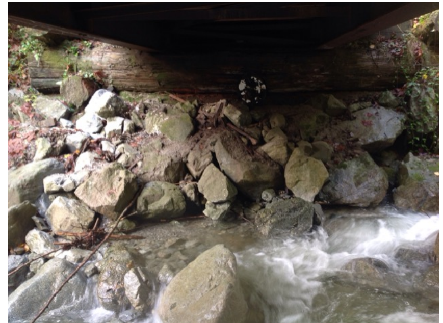
Right Bank Abutment when facing downstream
