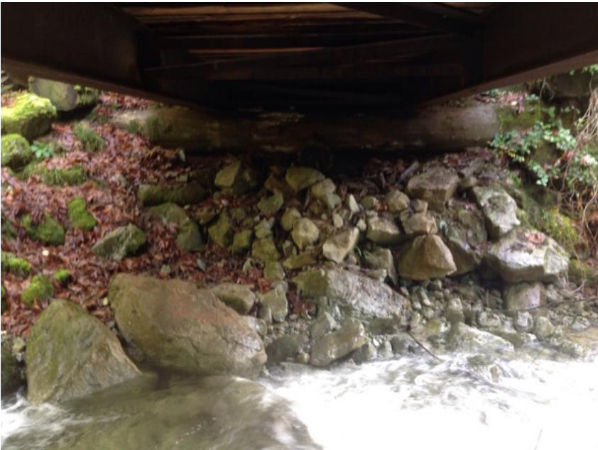
Left Bank Abutment when facing downstream
